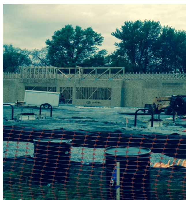
Framework for Casey's new Building
