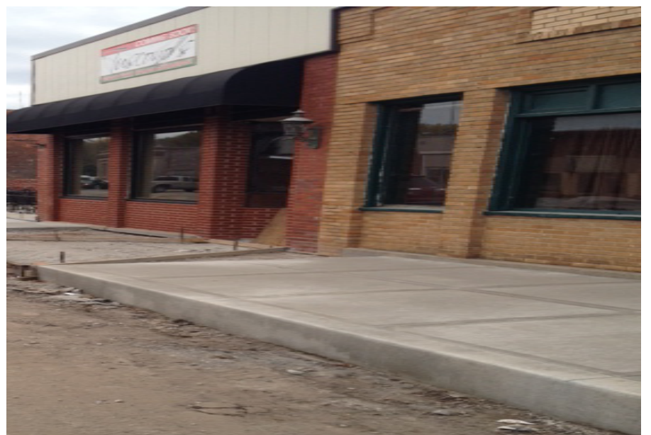
Pictured above are some of the newly laid sidewalks in downtown Buckner
