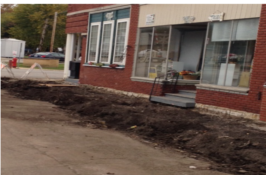
Pictured above is the ground work for laying the new sidewalks.
