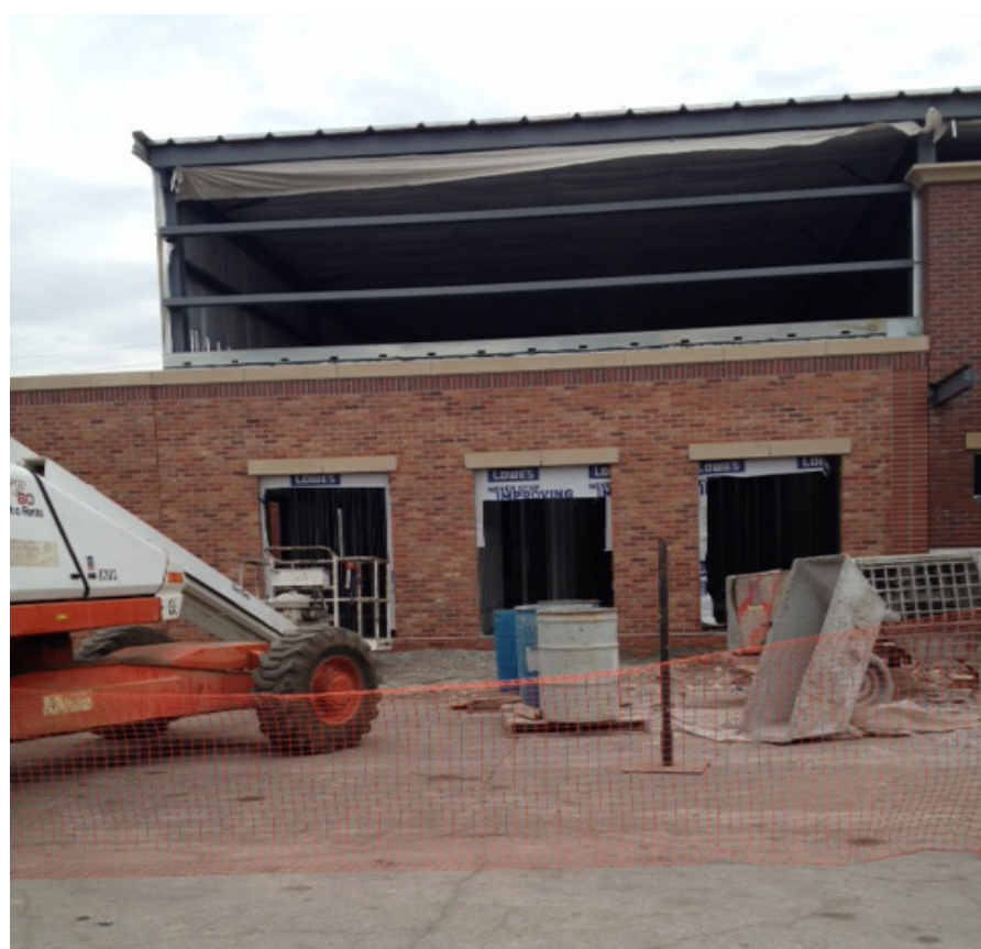
Pictured above is the new Buckner City Hall/multipurpose building on Hudson Street in Downtown Buckner. It's coming along nicely
