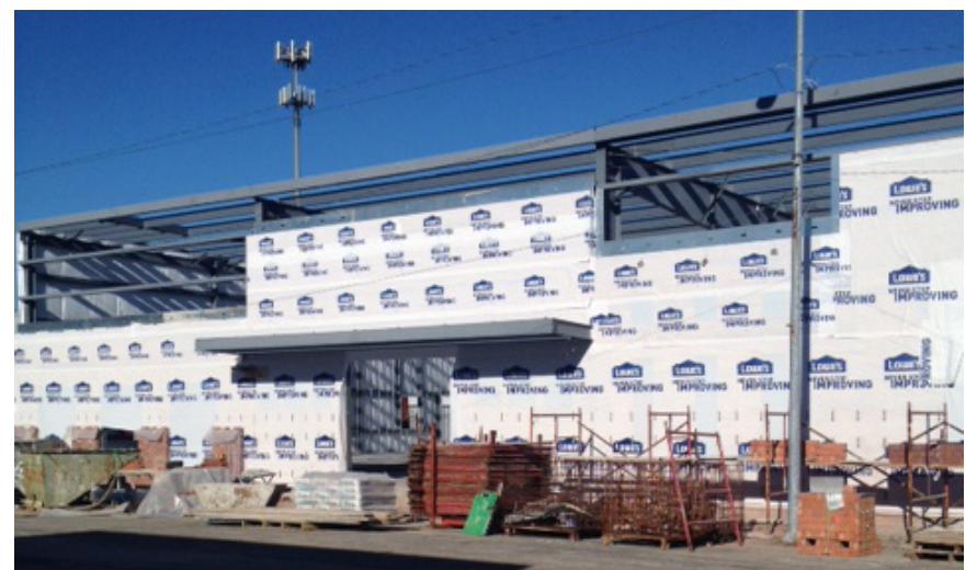
Pictured above is the new Multipurpose building, a work in progress.
