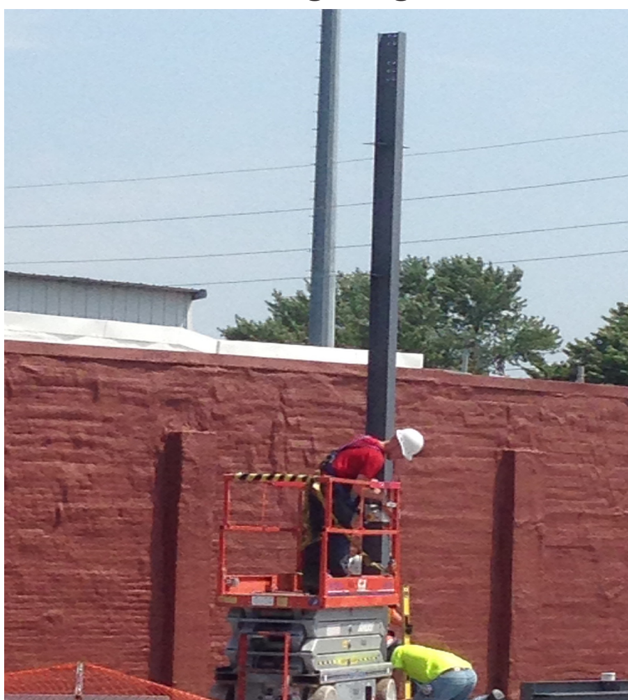
Pictured above is the first piece of steel being placed for the new multipurpose building. Thanks Kirk for the great picture!
