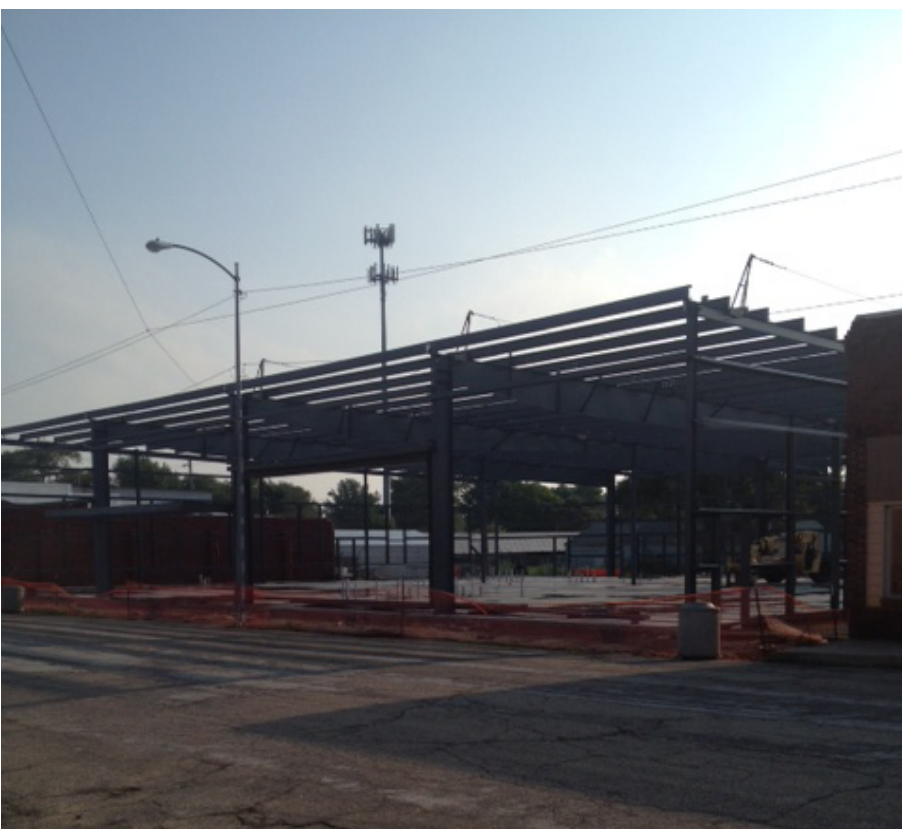
Pictured above is the new Multipurpose building, a work in progress.
