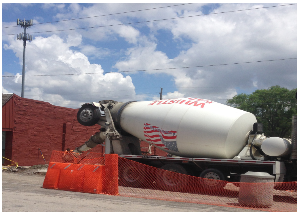
Pictured above is a concrete truck pouring the foundation for the new Buckner City Hall, located on Hudson Street in downtown Buckner. Thanks Kirk for the picture, paychecks in the mail!
